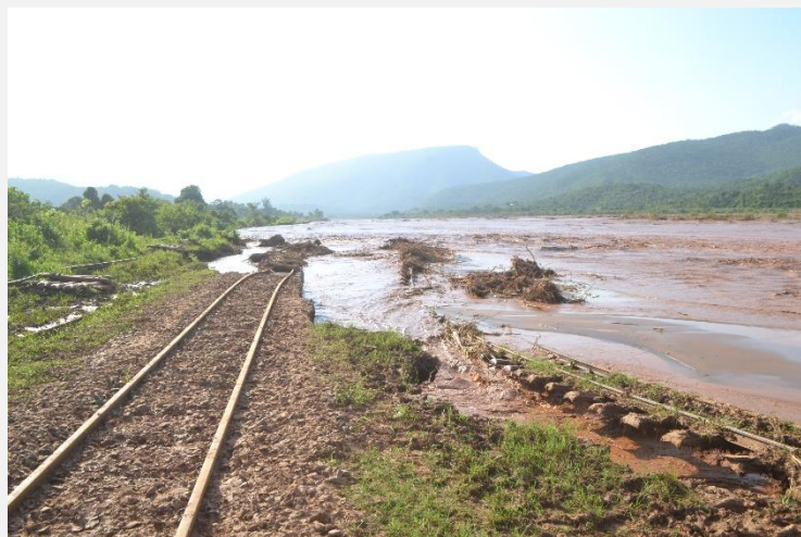
FIGURE 5-1: DAMAGE OF RAILWAY AT MUNISAGARA VILLAGE
