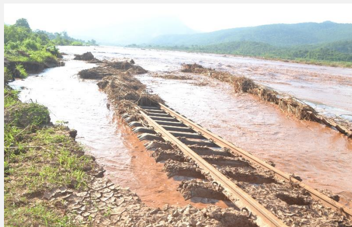
FIGURE 5-1: DAMAGE OF RAILWAY AT MUNISAGARA VILLAGE
